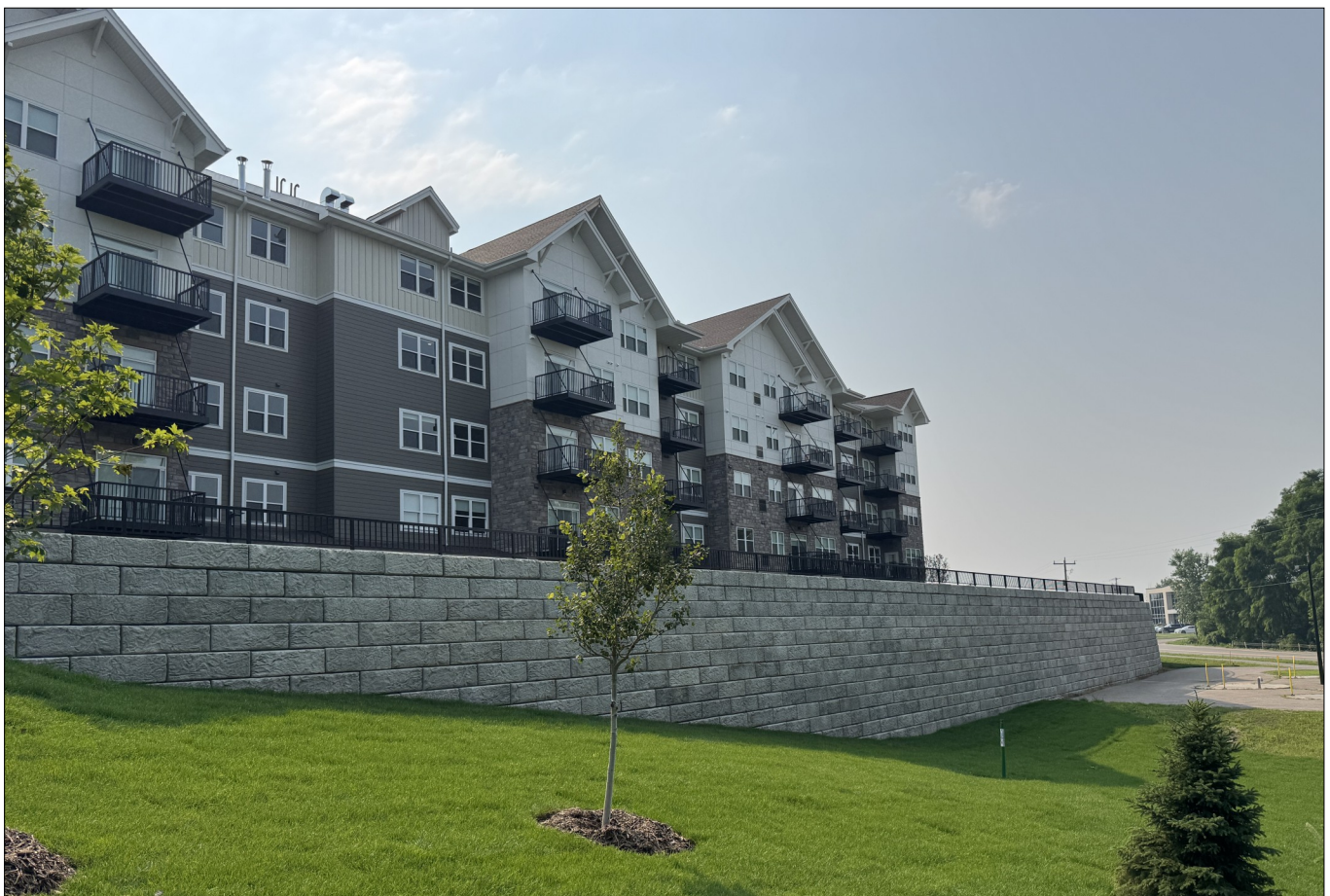
Photo 1 : View of Reinforced Soil Wall
