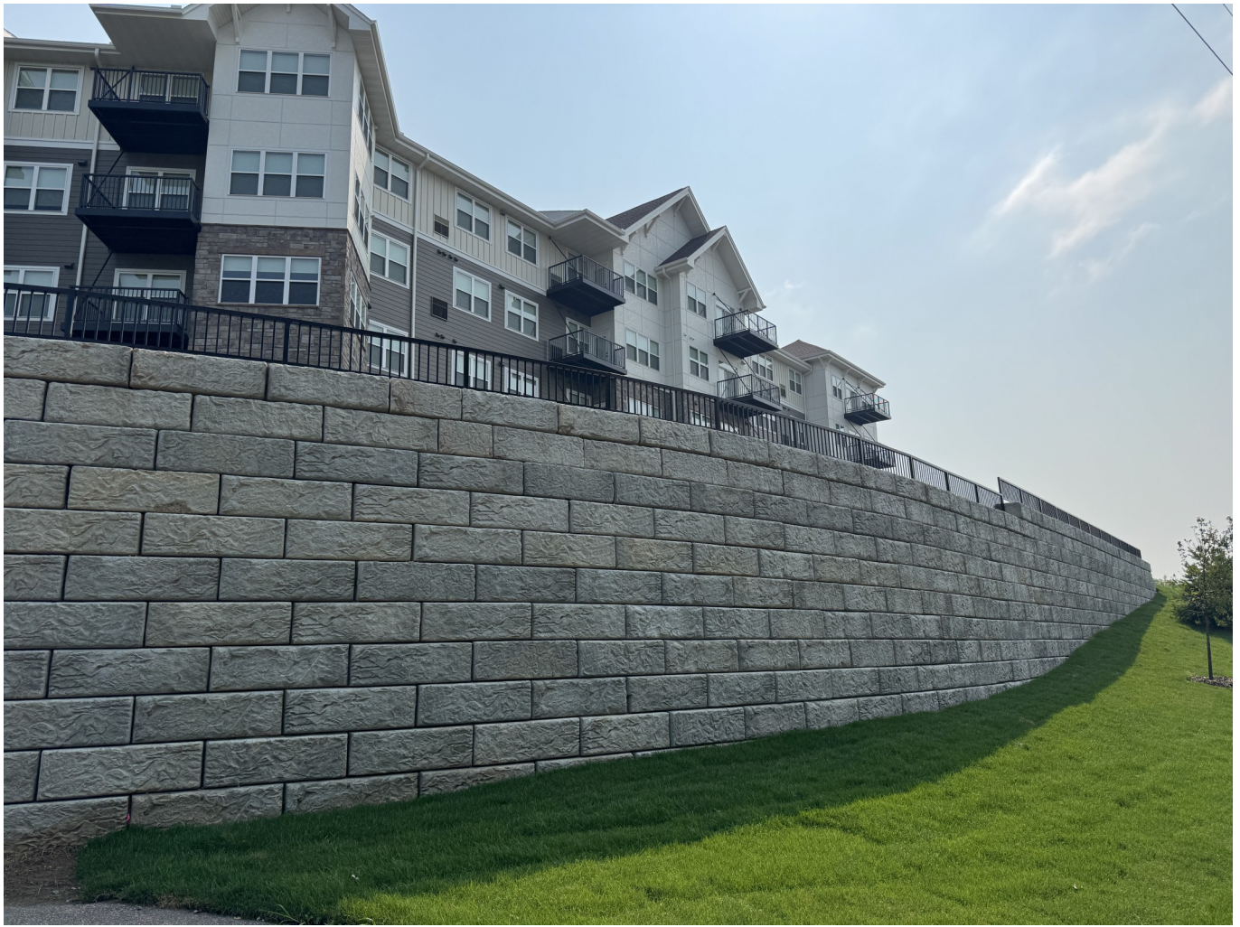
Photo 5 : View of Completed Reinforced Soil Wall
